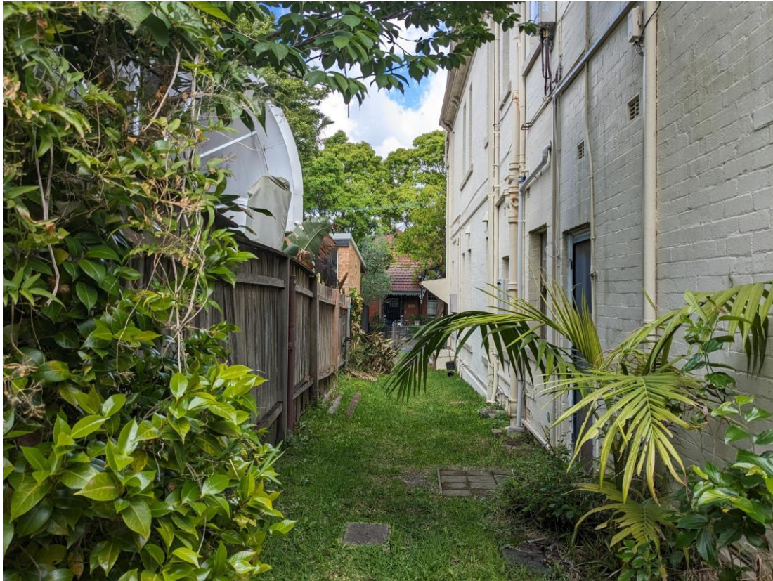
Figure 7: Open space/side boundary and southern façade viewed facing west
