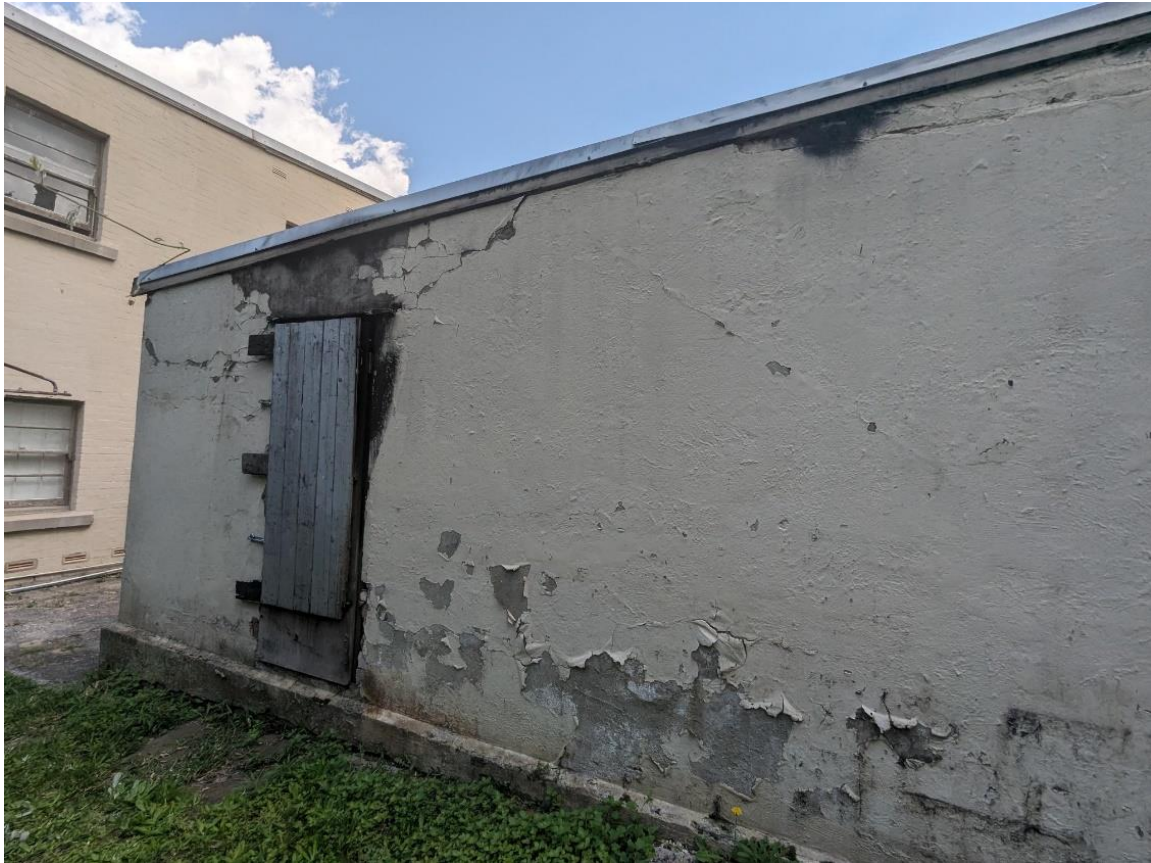
Figure 11: Existing garage proposed for demolition viewed facing north
