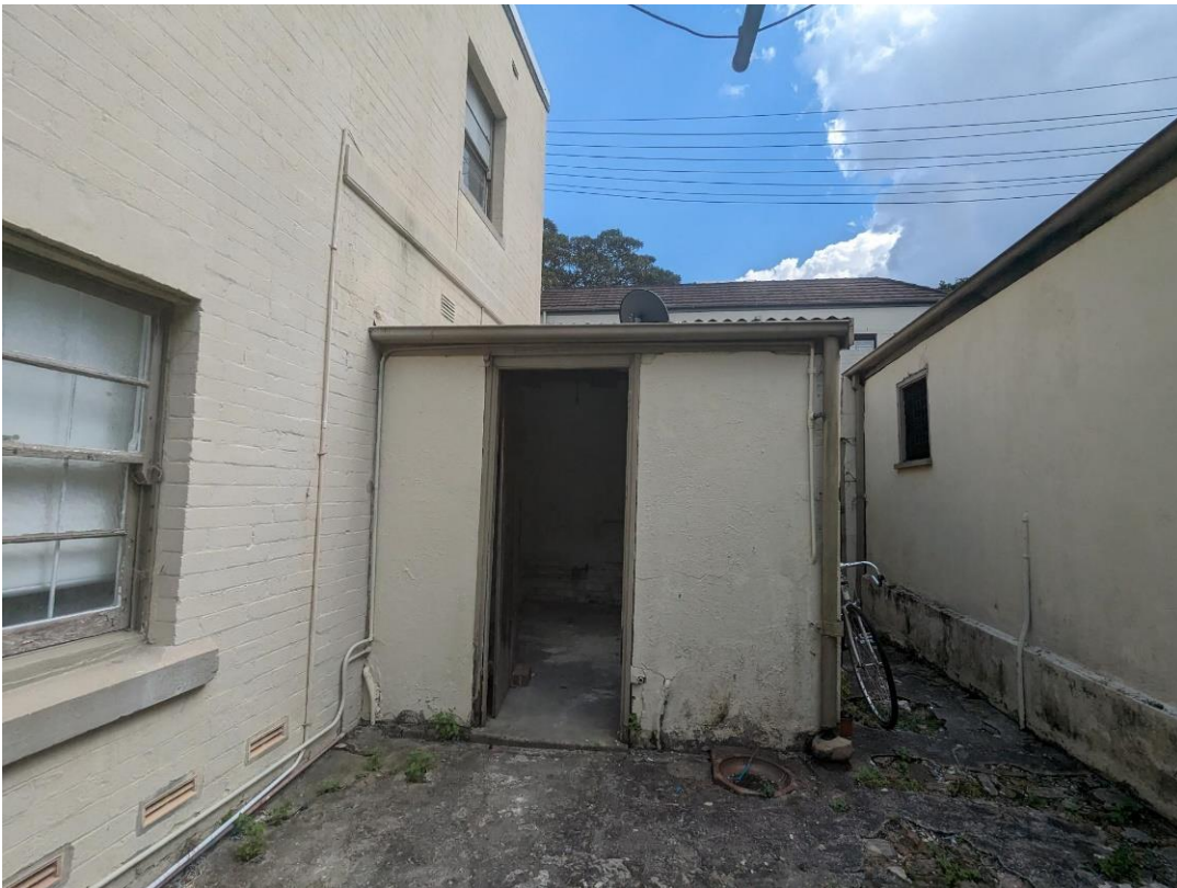
Figure 10: Existing shed/utility room proposed for demolition, viewed facing north
