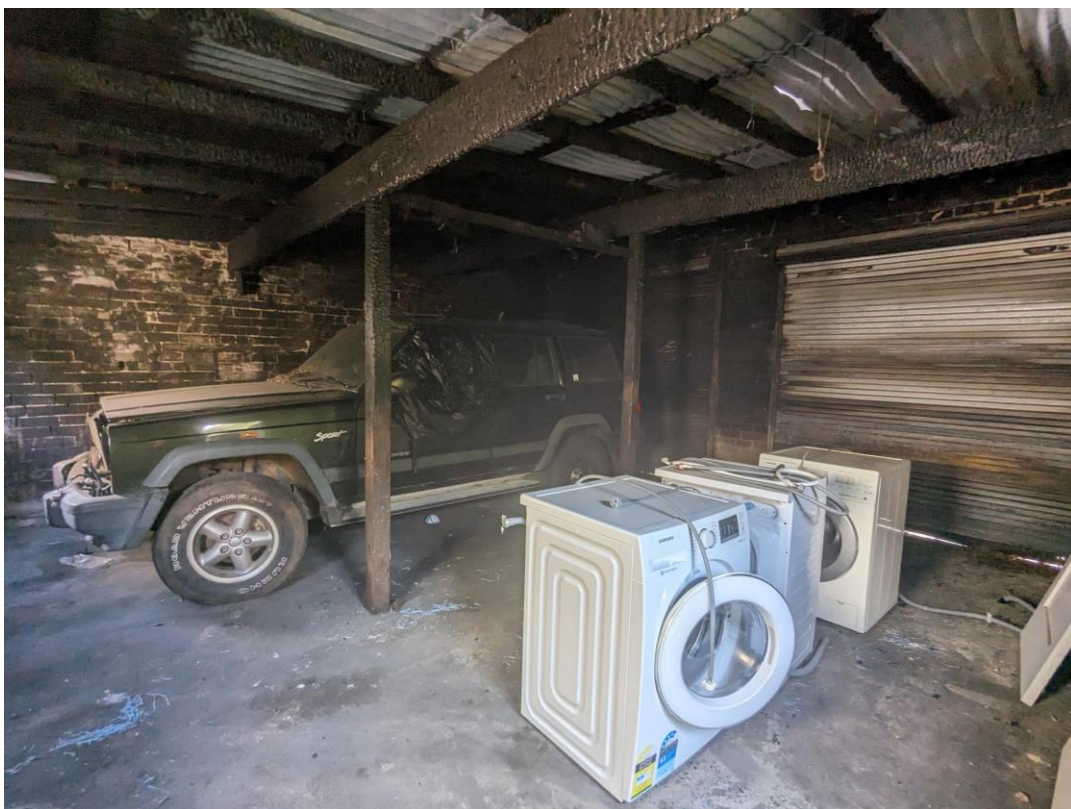
Figure 12: Interior of the garage proposed for demolition
