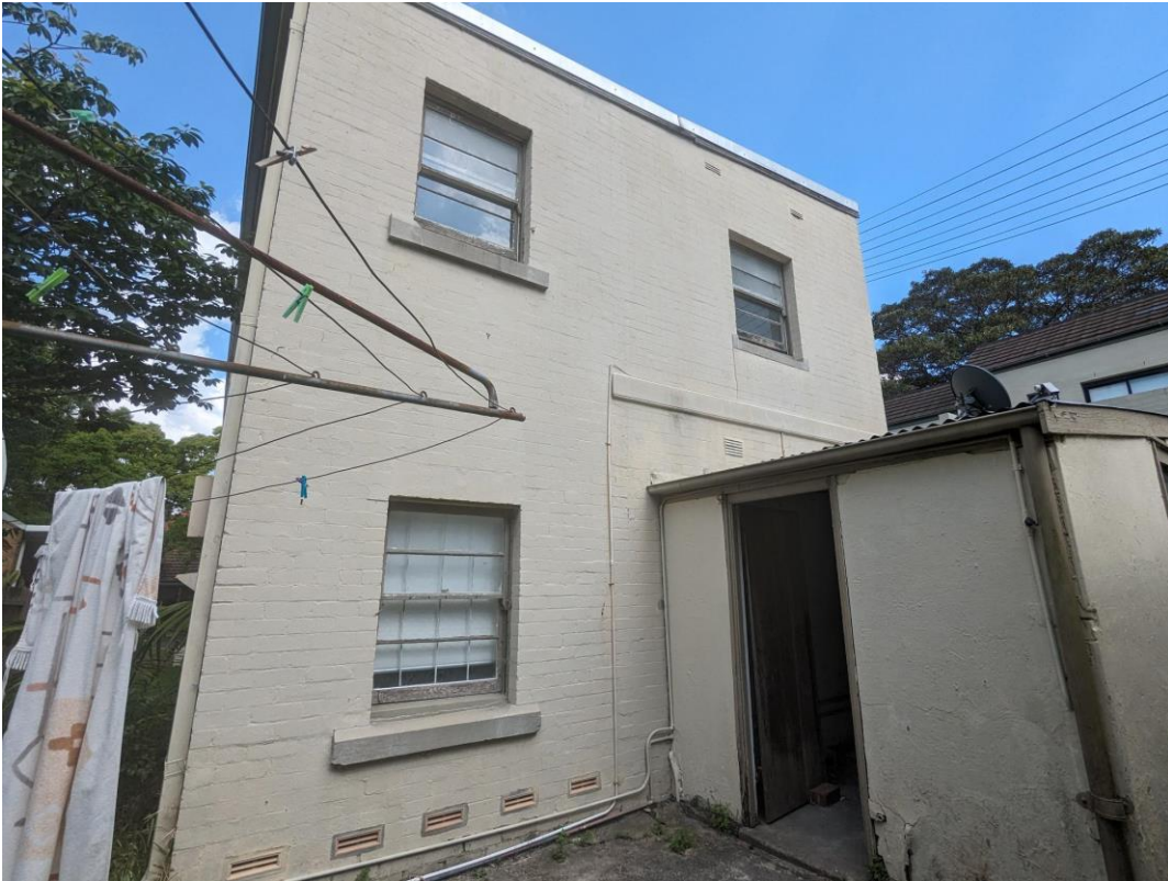
Figure 9: Rear of the existing apartment block and laundry/shed viewed facing west
